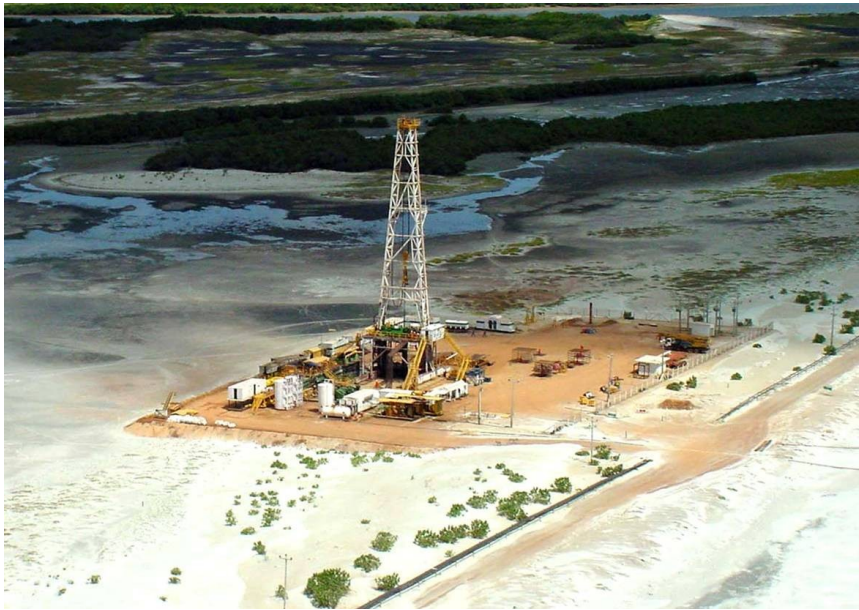
Fig. 1. Workover rig performing a maintenance service
