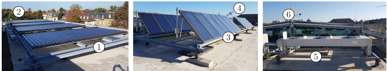
FIGURE 2 System components on the roof of the building: (1) vacuum tube solar collectors, (2) sensor T_{vtsc} , (3) flat plate solar collectors, (4) sensor T_{fpssc} , (5) recooling tower, (6) pyranometer and ambient temperature sensor
